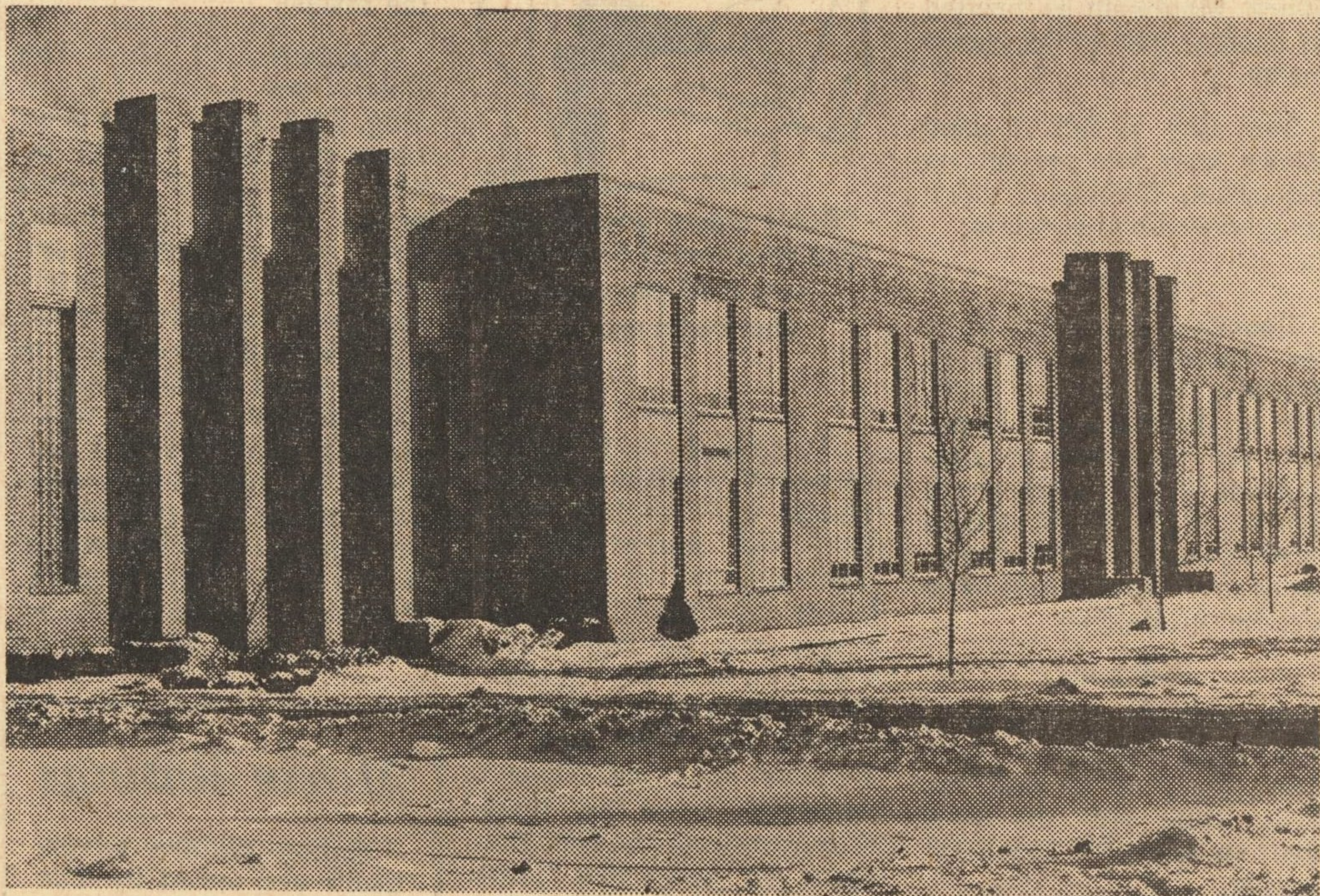
Johnny Appleseed Junior High School, opened in January, 1940, was built to serve the fast-growing south side of the city. The building cost $450,000, same as the John Simpson building, opened the same month and year. (Photos by Otto Schmidt.)
